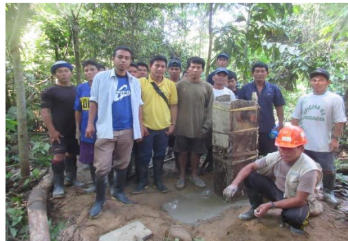
Teamwork for foundation of milestone 3 adjacent to Puerto Azul.
